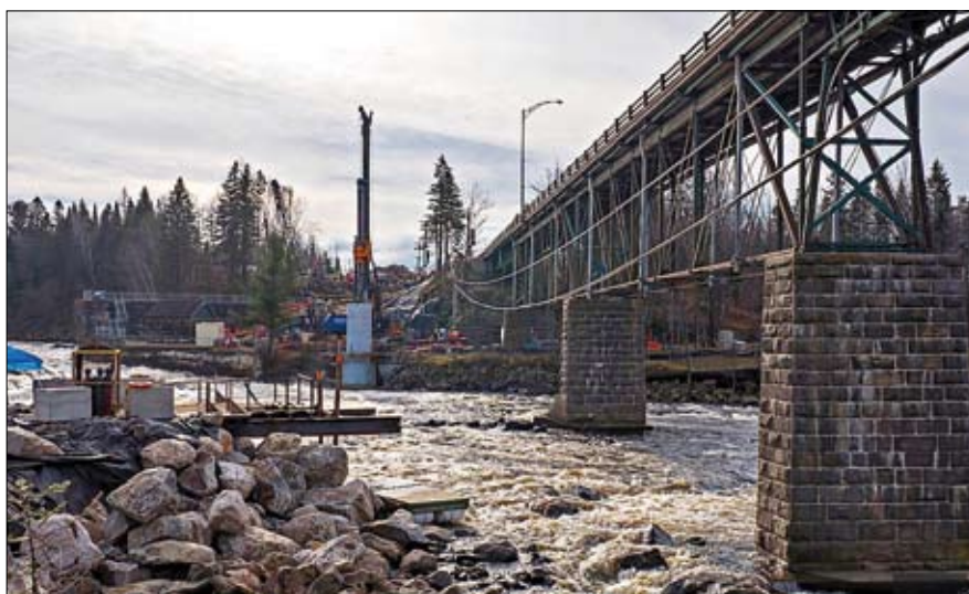
Delmag RH34 with SIP&T rotary tools during drilling operation
