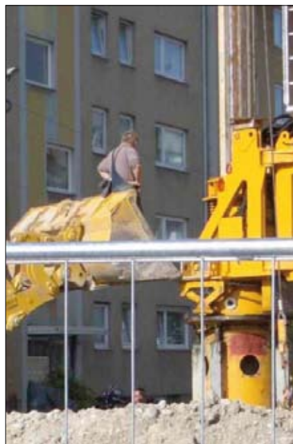
The use of a rubber loader as a "working platform" and safety harness are examples of inadequate means of access
