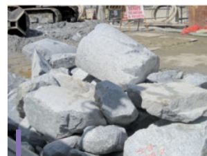
Pieces of rock extracted with the bored pile.
