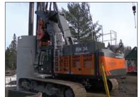
Delmag RH34 during drilling operation
