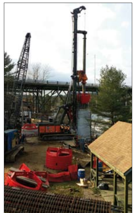
Delmag RH34 using Rock Bucket
